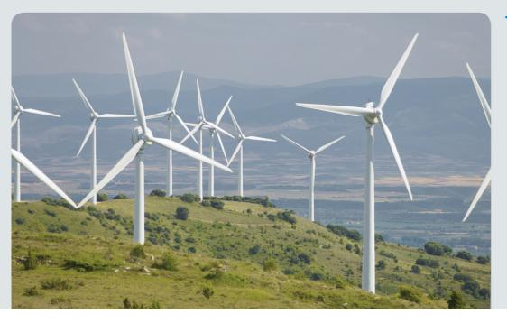
**Radius of wind** Power output turbine arms (m) (MW) 70 1.5 80 1.8 90 3.0 120 4.1 190 11.0
